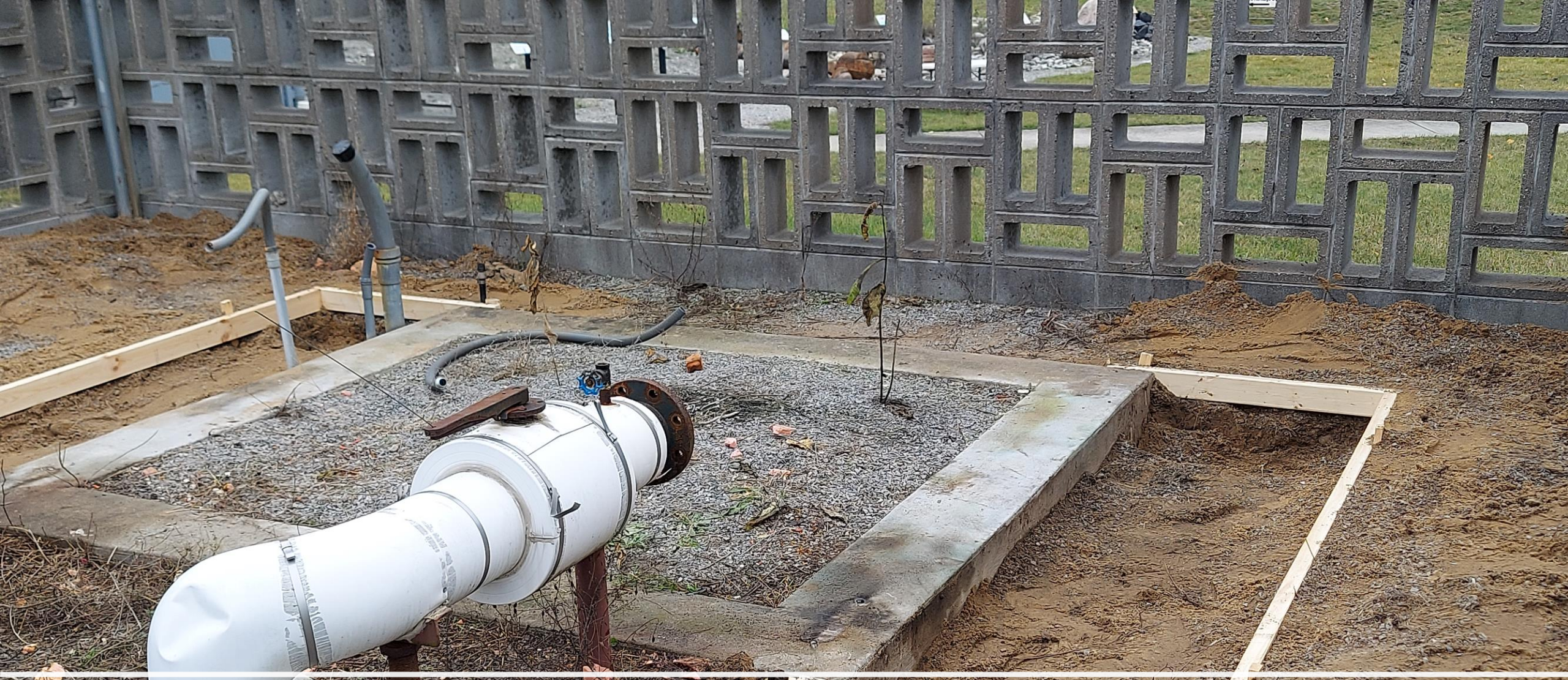
The new foundation framed for the chiller. Along with the old electrical conduit.
