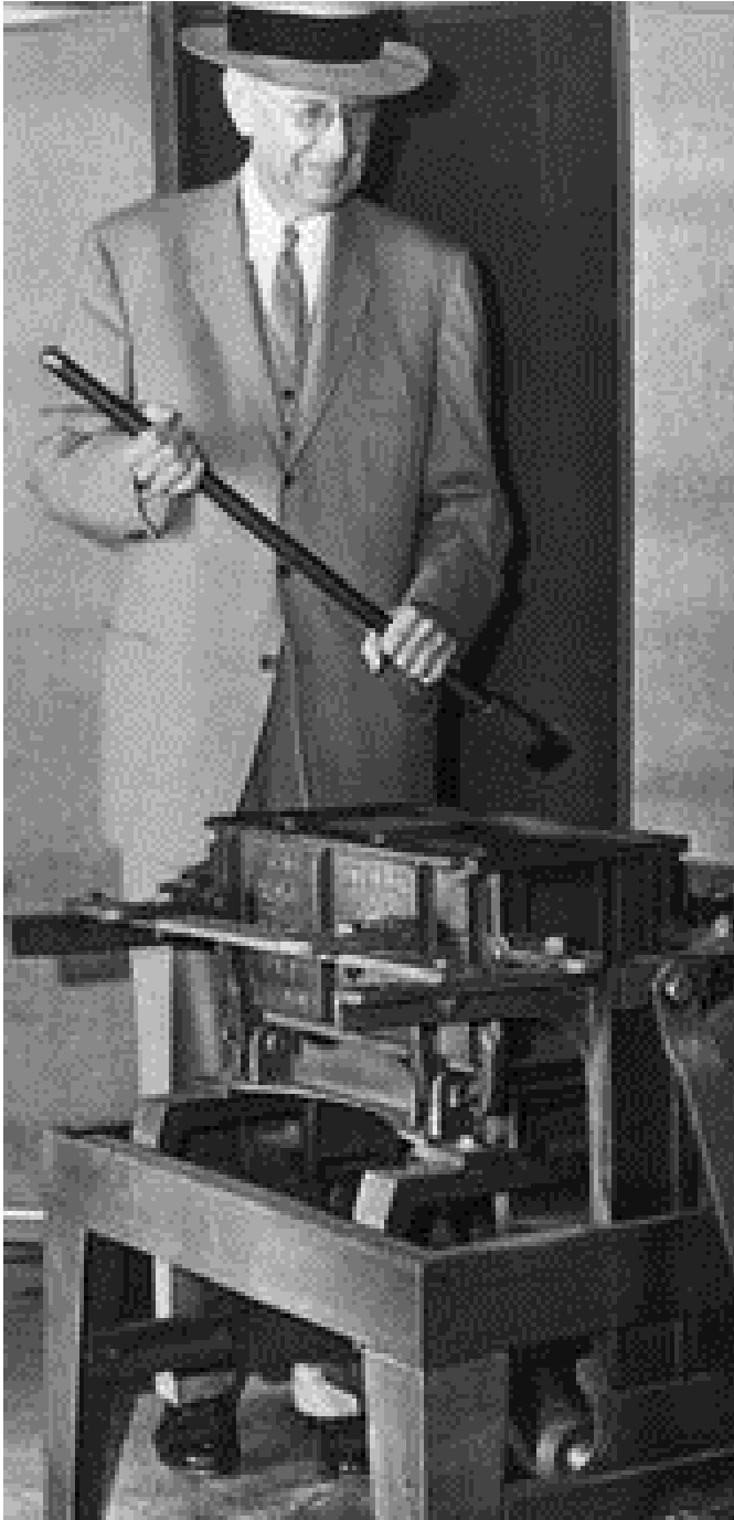
Founder Jesse Besser with one of his company's first hand-tamp block machines produced in Alpena. A similar machine is on exhibit at the museum.
